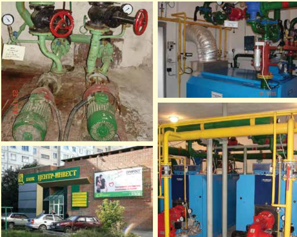
Fig. 2.11. Equipment modernisation freed up premises for a Center-invest Bank office.
